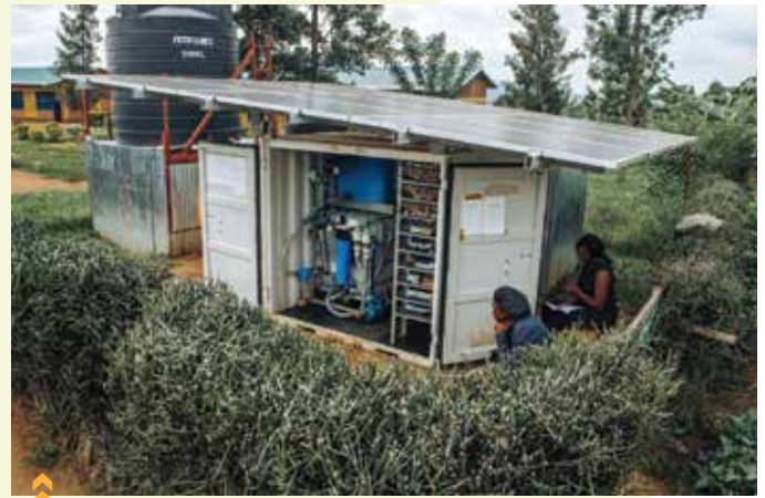
OffGrid Box with Solar Panels on the Roof
